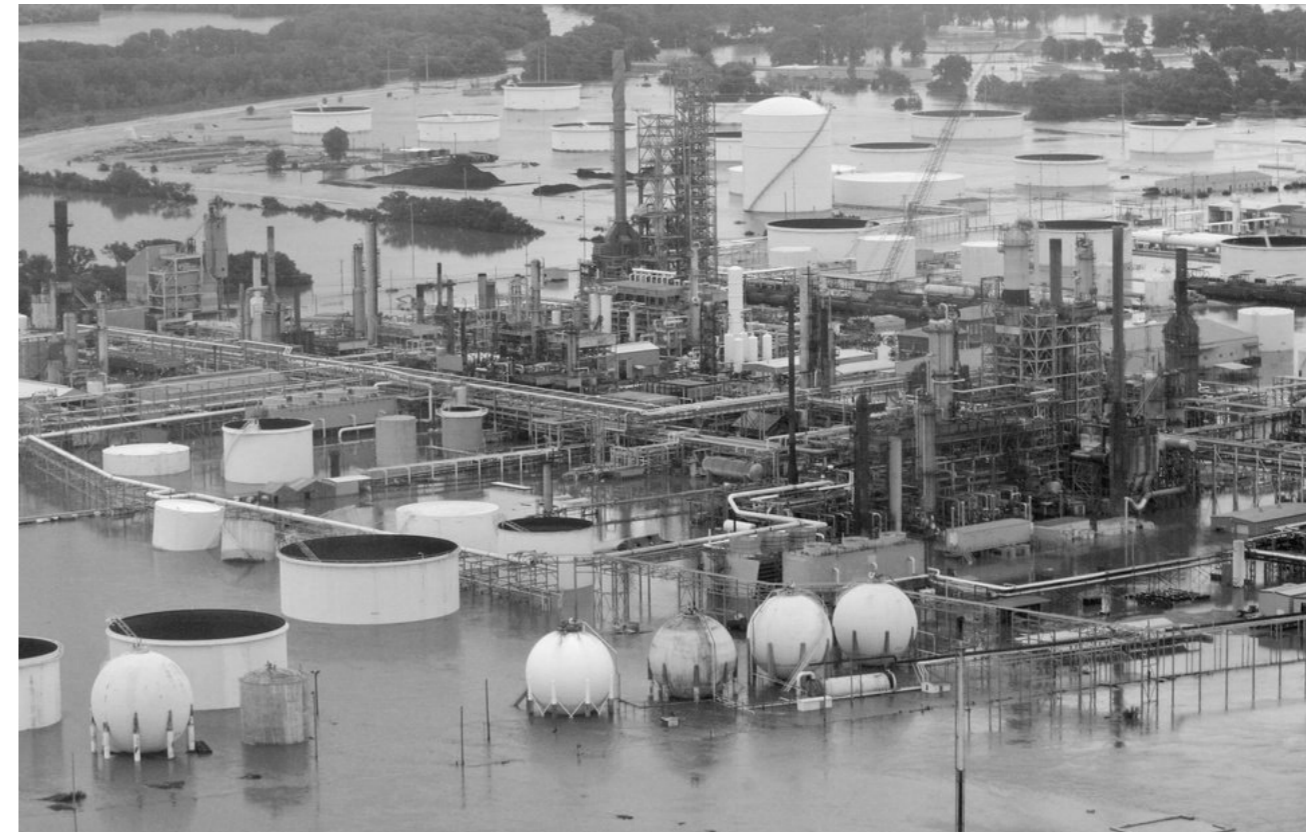
Figure 8: Coffeyville refinery flooding. Source: Orlin Wagner.
