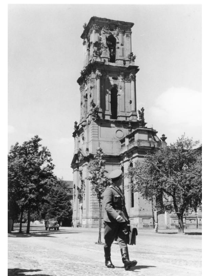
17. The damaged bell tower of the Garnisonkirche during the time of the GDR. 1960
