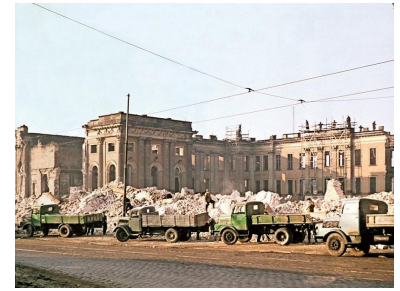
11. Demolition work on the Stadtschloss. Estimated 1960
