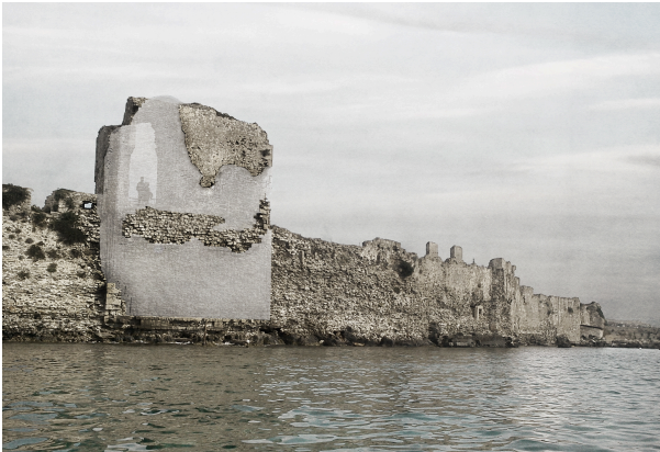
Figure 1. Illustration of the cast glass masonry
