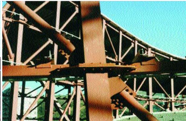
B. Connection between two column segments and bracings.
