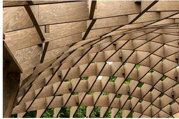
B. Change of direction in the roof structure (Olll-Architecture-Gallery 2005).
