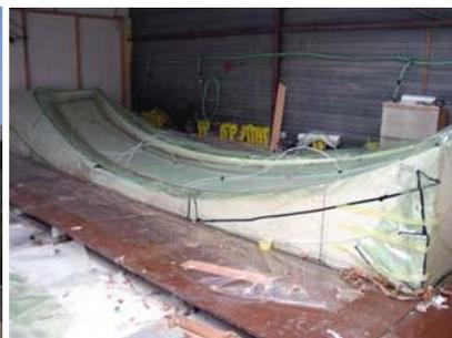
B. Vacuum injection of the exterior surface of a shell segment.
