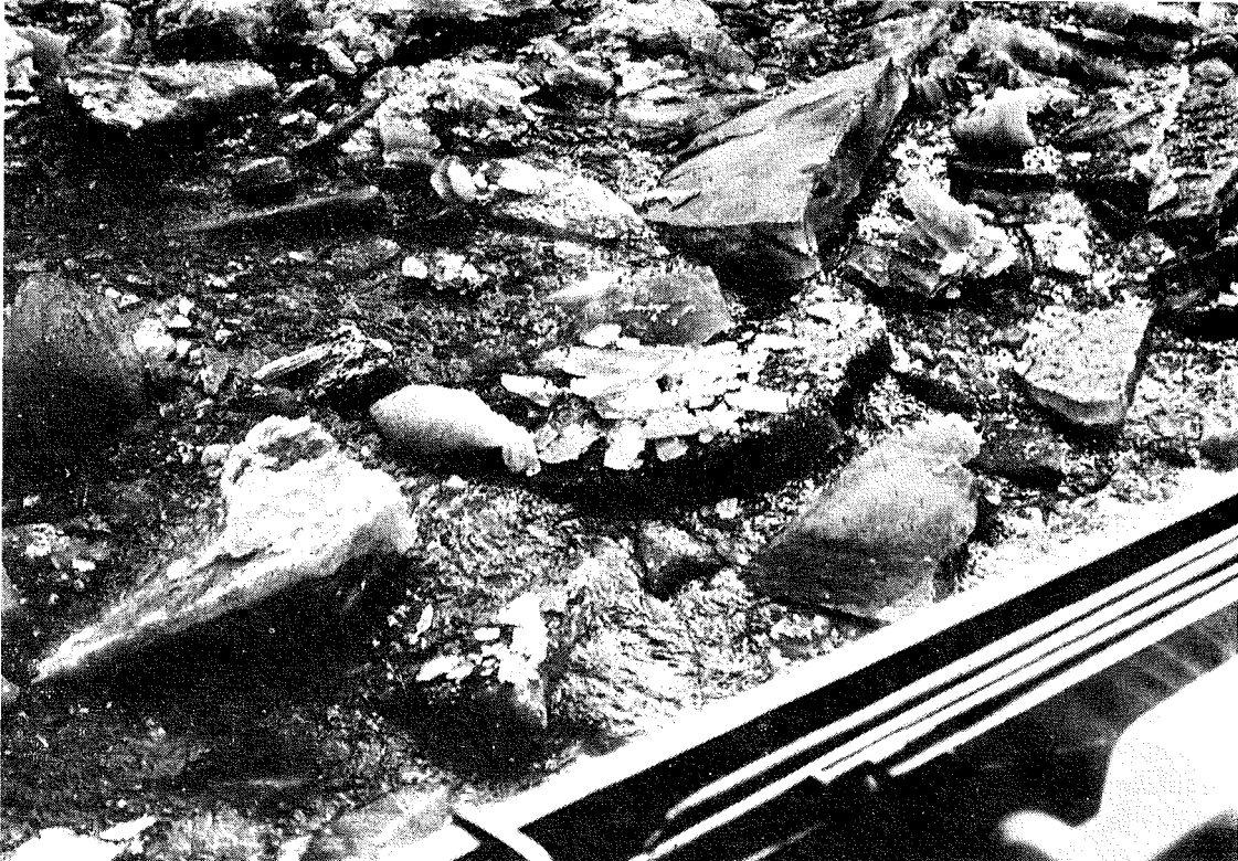
Ice floes slid underneath each other at Hardinxveld on the Upper Merwede, February 1929. The ice-breaker (part of which is to be seen in the right lower corner) is steaming backwards. Ice floes shooting to the surface.
