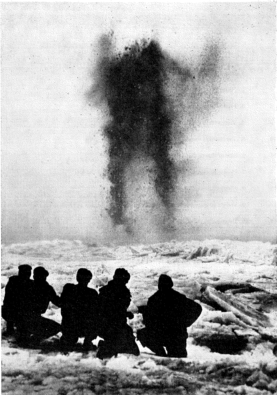
Clearing ice barriers with dynamite.
