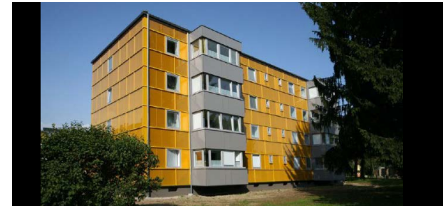
East-block facade renovations energy cost reduction
