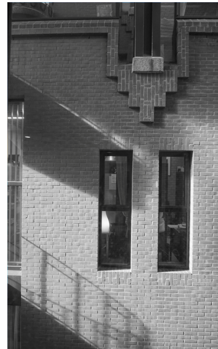
Existing Facade Composition
