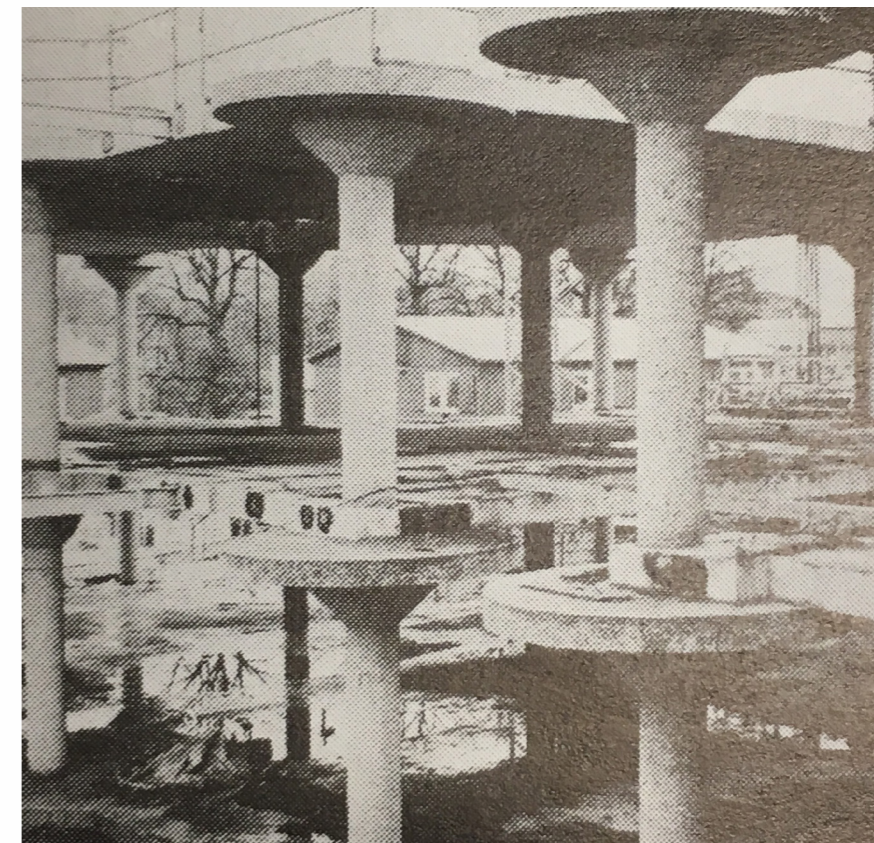
Reinforced concrete structure of Humanities Faculty Buildings in 1981 - Cement XXXIII
