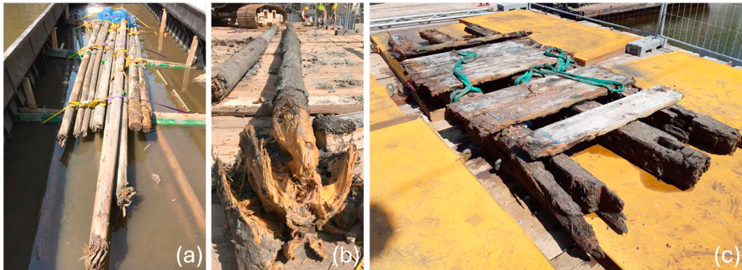
Fig. 1. (a) batch of timber piles extracted from Bridge 30; (b) broken tapered end of the pile due to the effect of biological decay and compressive load; (c) part of horizontal foundation of Bridge 30.
