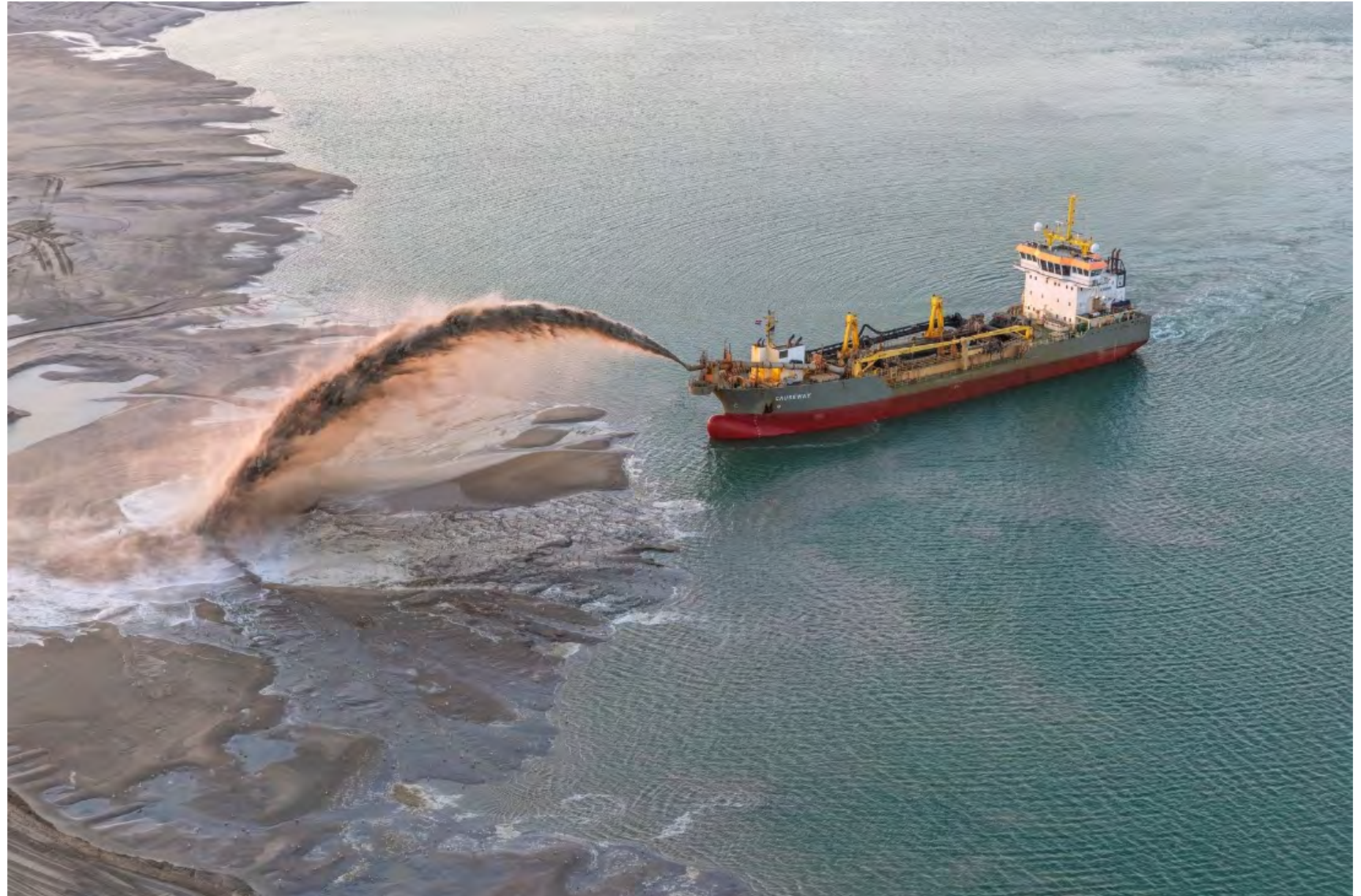
Replenishments, dredging and pumping sand onto beaches. Photo: Zlatan Hrvacevic, 2022.
