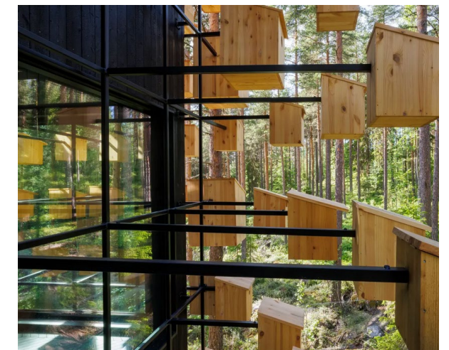
Figure 51 and 52. Close up images of the Biosphere where the connection between the façade and bird houses is visible. (Source: BIG, 2019)
