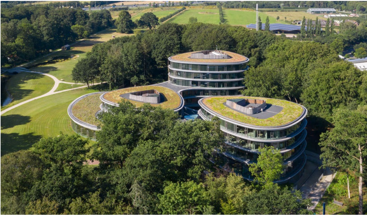
Figure 44. Top view of the Triodos Bank (Source: RAU Architects, 2019)
