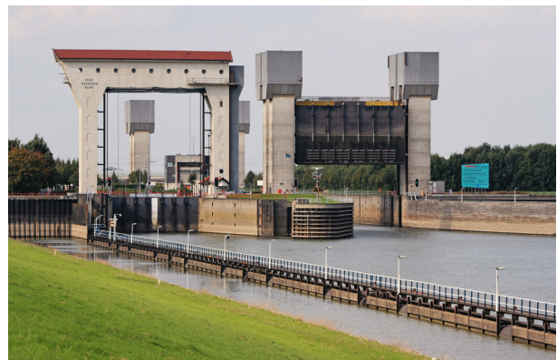
Figure 14: Illustration of a Vertical Lift Gate and Vertical Lift Gates at the Prins Bernhard Sluis [NLD]
