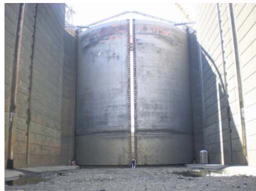
Figure 16: Right: Illustration of a Mitre Gate, Left: Arched Mitre Gates of the Dallas L&D, [USA]
