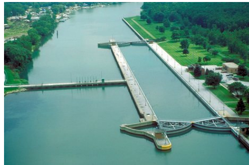
Figure 21: Right: Illustration of a Sector Gate, Left: Segment Gate of the The T.J. Obrien L&D, USA
