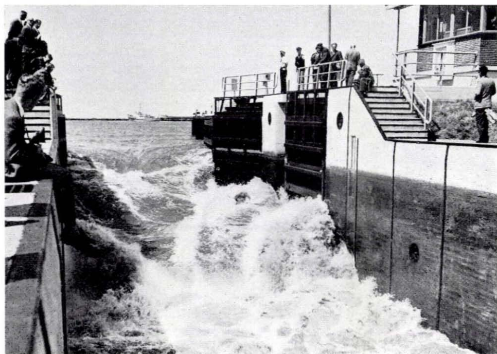
Figure 11. Idem: the wing-gates almost completely open.
