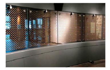
achieved by shifting a series of fritted glass layers, aligning or diverging the pattern.
