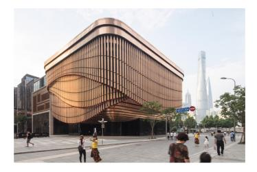
The building has been inspired by the traditional Chinese theatres. Its envelope is made by three layers of bronze tubes that work as shading system all around the building. According to the direction and amount of daylight, the three layers adjust their position changin the level of transaprency of the facade. The effect is a dynamic envelope that seems to rotate around the building is a very fluid effect.
