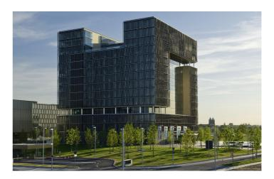
The building has two facade typologies: two fully transparent that act as gigantic windows and the rest that is covered by triangulr panels made of stainless steel lamellas. The latters, change orientation by rotating horizontally according to the sun position and, thanks to the lamellas, they redirect the light without blocking the view. When the triangular panels are perpendicular to the facade, the orthogonal view is completely free from obstructios.
