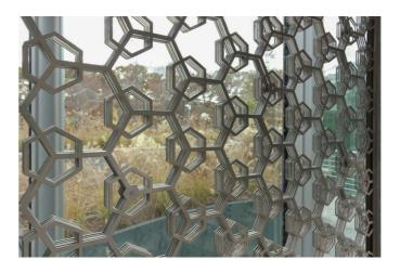
The installation in Simon Center shows three possible artistic patterns for a dynamic shading system. The geometry has been designed in a way that three layers with the same geometry can shift from an overlap position to three different positions that create different patterns decreasing the amount of transparency. By this way, the system regulates daylight and solar heat gain, decreasing the energy demand needed for cooling during summer.
