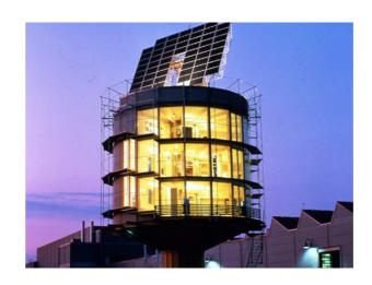
Heliotrope is one of the first zero-energy houses in the world. It is mounted on a pole that allows it to rotare of 180 degrees during the day, taking advantage of the sun radiation, increasing the amount of daylight into the indoor space and assuring heat gain thanks to the solar thermal pipes on the facade. The PV panels and the solar thermal tubing provide both electricity and heating, transforming the project in a perfect example of sustainability.
