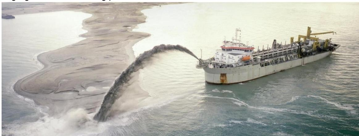
**Figure 1.1 Hydraulic placement rainbow method**
