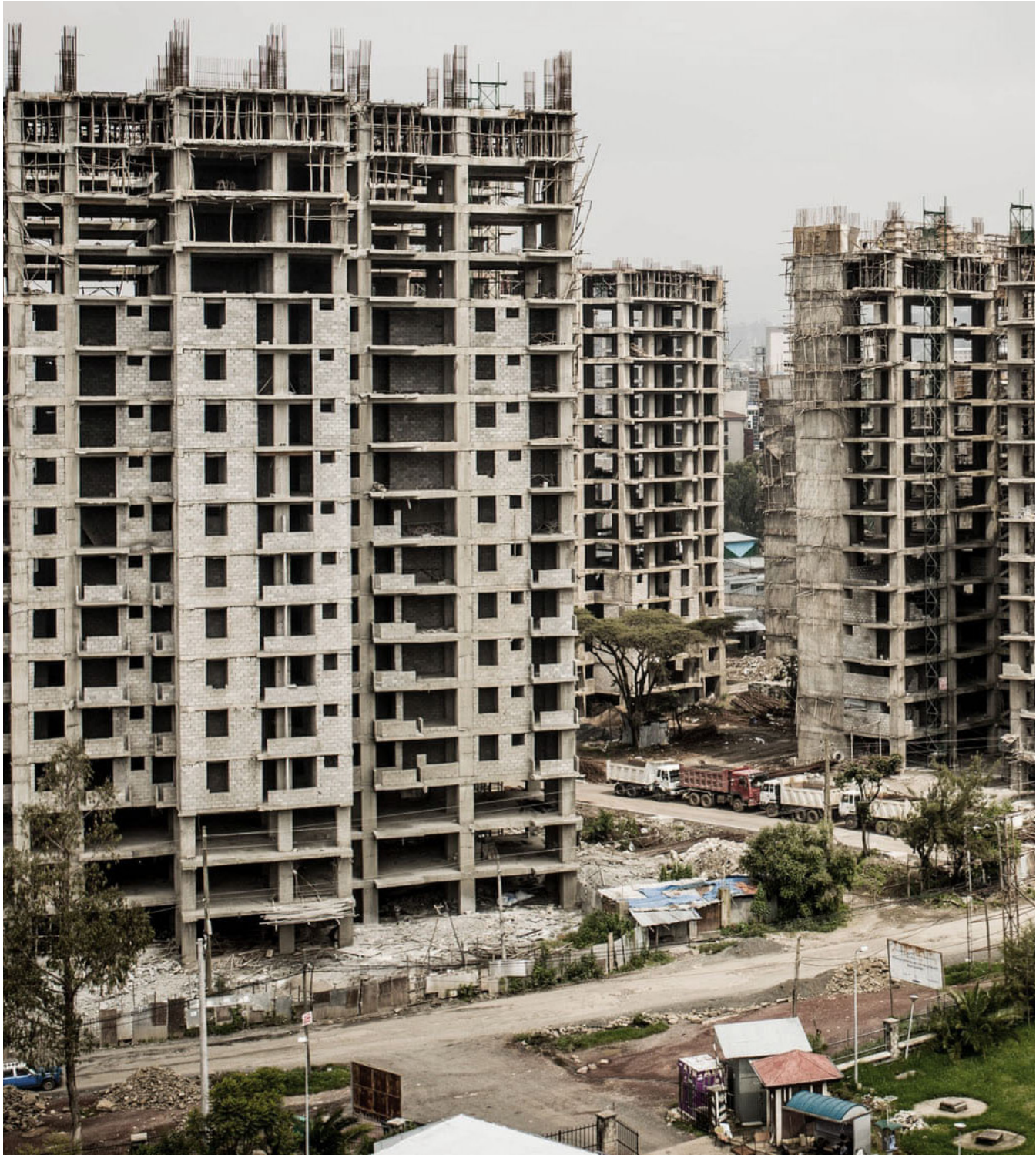
Condominium construction site
