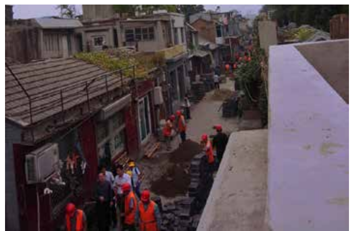
Figure 121. The construction has begun in 2012; renovation of the pavement and buildings.
