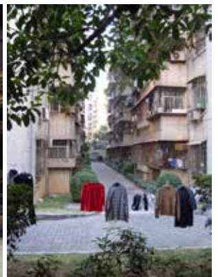
Figure 82. Liyuan village consists of multiple large dormitories and apartments protected by walls and gates.
