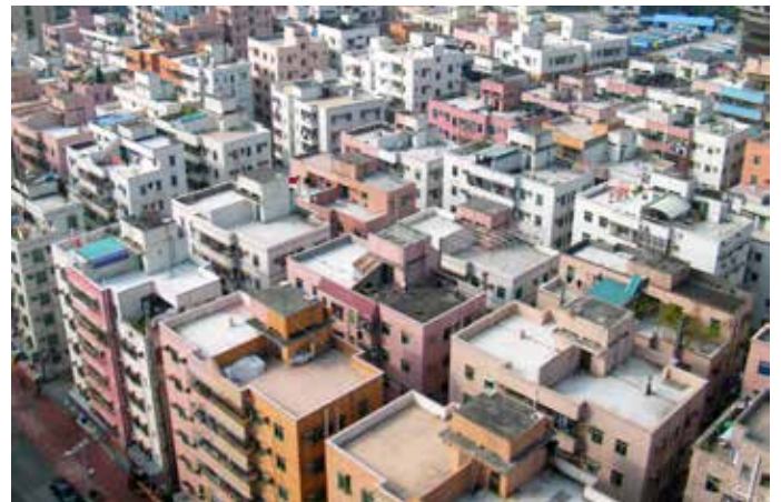
Figure 55. Majority of houses in an urban village have a plot of 10 by 10 meters. In some cases the owner expands towards the neighbouring house, creating so called Handshake buildings . Some owners build as many as 12 storeys without formal permission. Shui Wei urban village (O'Donnell, 2012).
