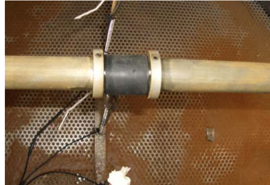
Figure 6-9 Test 1, the rubber sleeve is closely connected to the steel blockade rings
