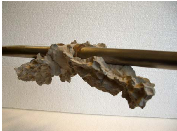
Figure 6-45 Side view of the grout fracture
