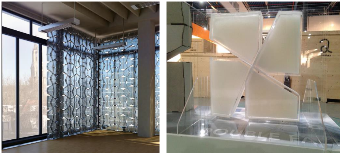
Figure 1. Artist impression and photo of the first adjustable translucent Trombe wall prototype.
