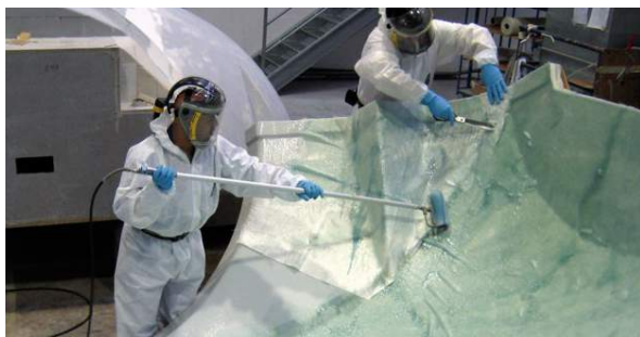
6.2 Operation of hand lay-up ( http://www.fassmer.de )
