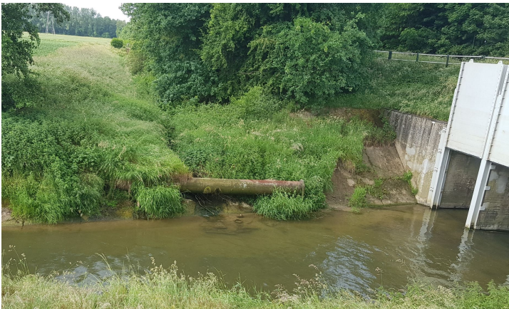
Figure B.1: Picture of the seepage stream
