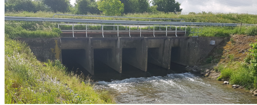
Figure 4.1: Outlet of the inverted siphon
