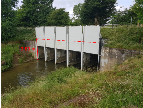
Figure 1.4: Inlet of the inverted siphon (own picture).
