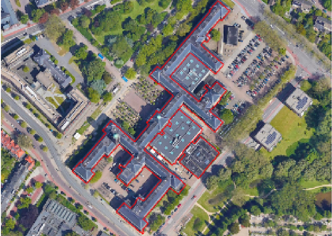
Figure 3.4.: Visualization of Bouwkunde (Faculty of Architecture and the Built Environment).
