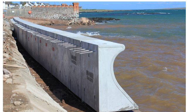
Figure 9.3: Bull nose at the Donaghadee sea wall (UK). Source: www.moore-concrete.com
