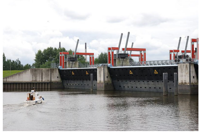
Figure 9.9: Large hydraulic valves in Hamburg. Source: http://www.bildarchiv-hamburg.de
