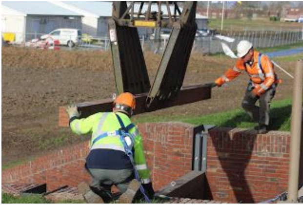
Figure 9.8: Placement of stop locks. Source: hanviskie.blogspot.nl
