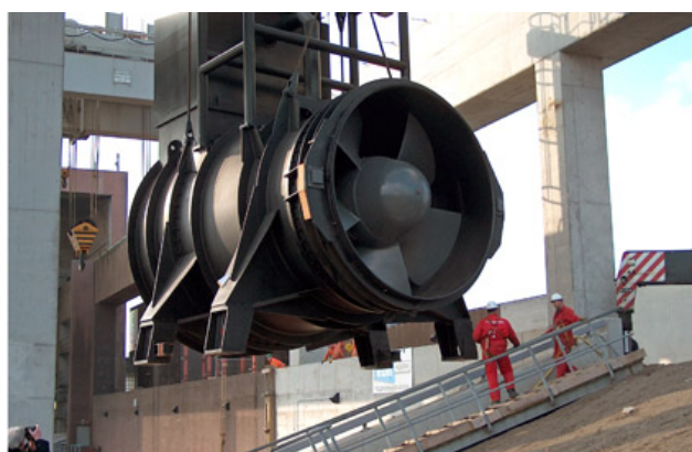
Figure D.1: Conventional pump (IJmuiden). Source: www.gemalen.nl
