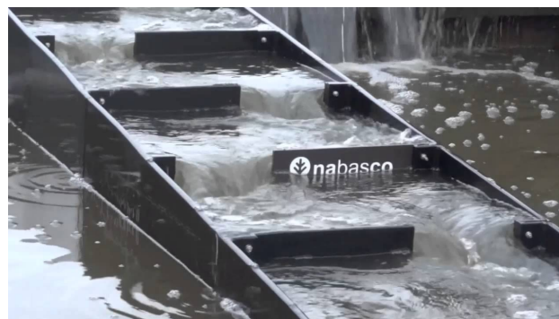
Figure D.5: Baffle fish ladder. Source: www.youtube.com
