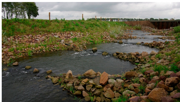
Figure D.4: Pool-and-weir fish ladder. Source: www.wrij.nl
