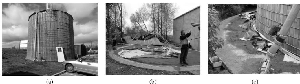
Figure 3. Timber stave water tanks: (a) typical tank c. 1980s; (b) collapsed tank; (c) damaged tank (courtesy FPANZ).
