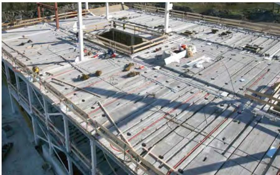
Figure 1. Erection of precast hollowcore slabs in a floor structure of a building.
