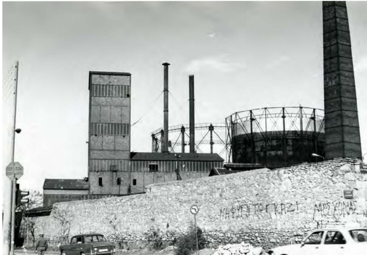
133. The gas factory at the mid 20 th century. Source: Adrakta et al. (2005)
