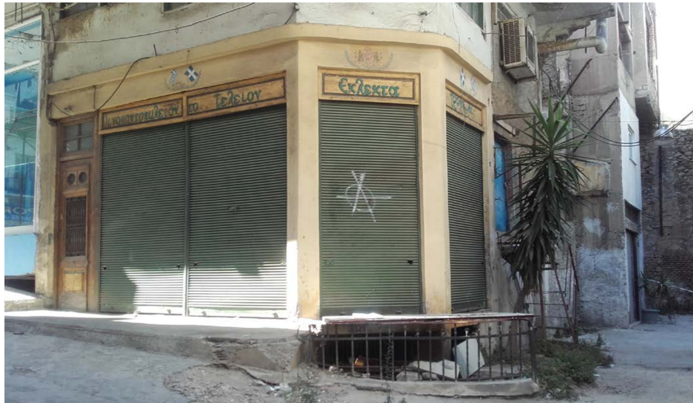
53B. Typical store with items of everyday use. It is representative of the daily routine that used to take place in the commercial/industrial area of Agios Dionysios neighbourhood in Piraeus. The original labels, the door and windows are preserved. Photo by author.
