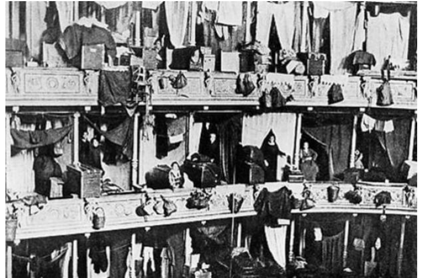
28. The municipal theatre of Piraeus used as temporary refugees accommodation. One balcony per family which would soon transform into self-constructed houses, places that people would call home. Source: http://www.lifo.gr/team/lola/60328
