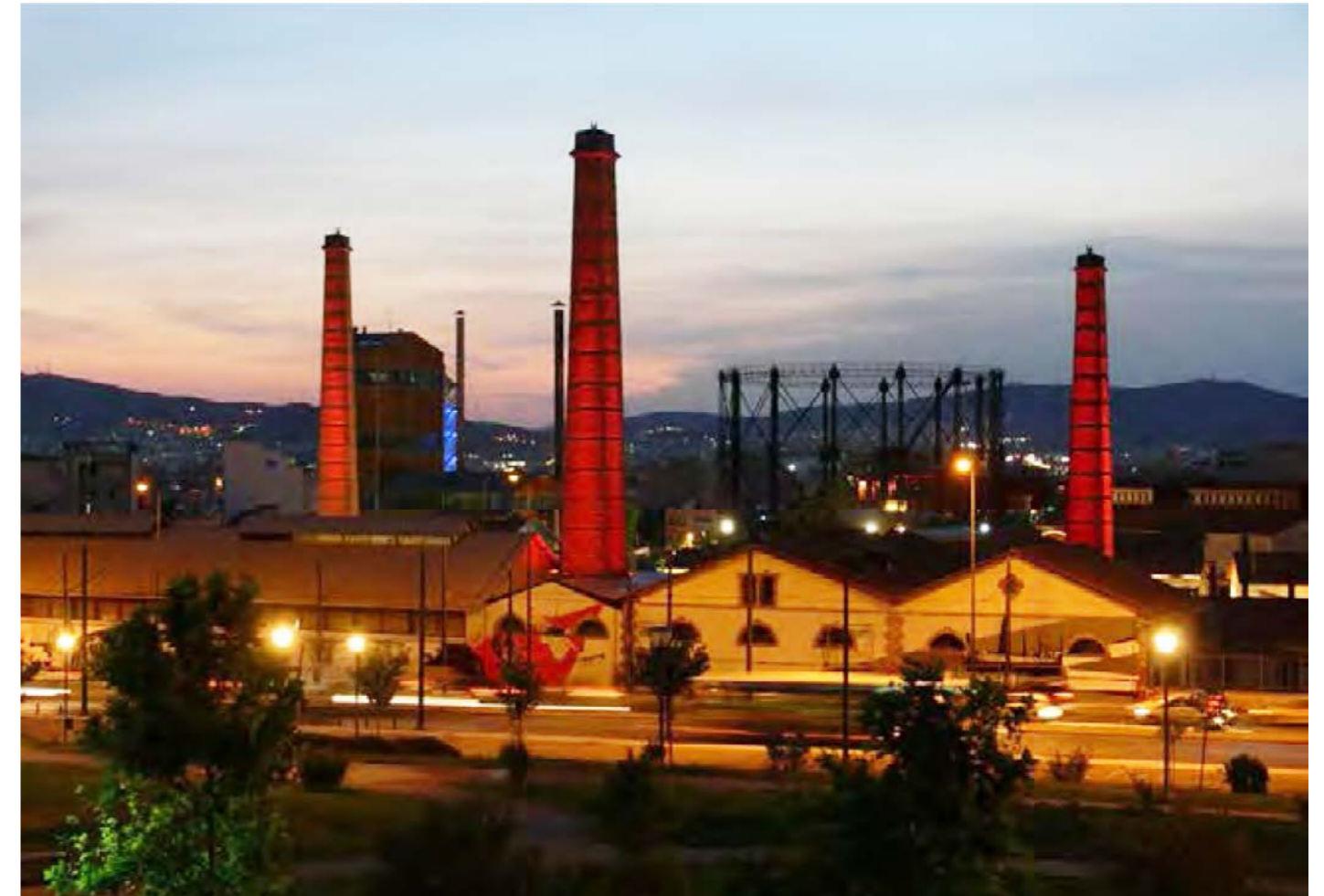
135. Technopolis Gazi- centre for culture and technology. The old factory after the renovation has become a famous destination for nightlife. The area around hosts from alternative theaters and underground bars to pop music scenes and fancy clubs. Source: Adrakta et al. (2005)
