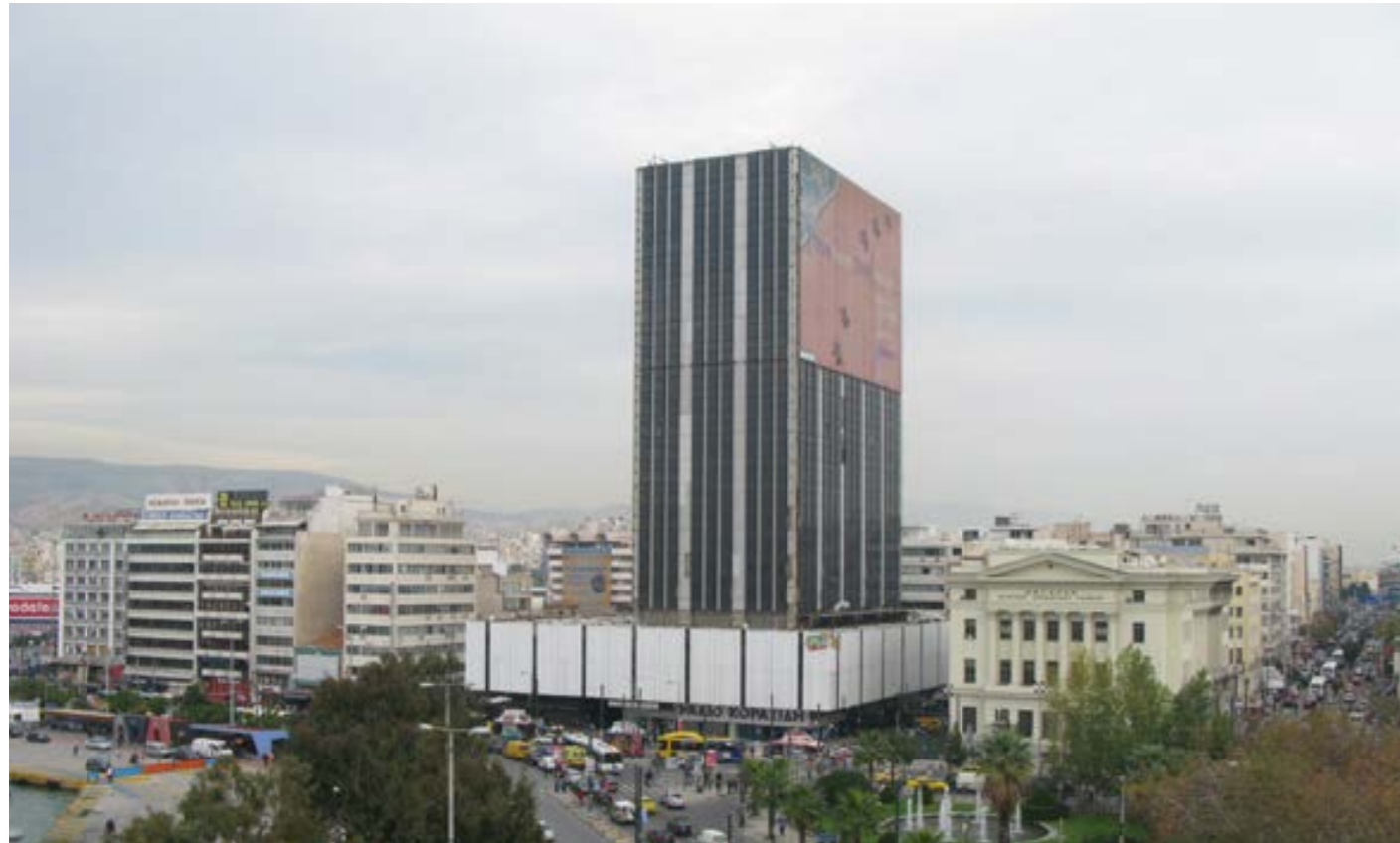
53A. The Tower of Piraeus ; one of the few skyscrapers in Athens (and Greece overall), built in 1972-1983. Only the first three floors have been ever used. The rest remain empty until today, for various reasons. Source: http://www.greekarchitects.gr/gr/
