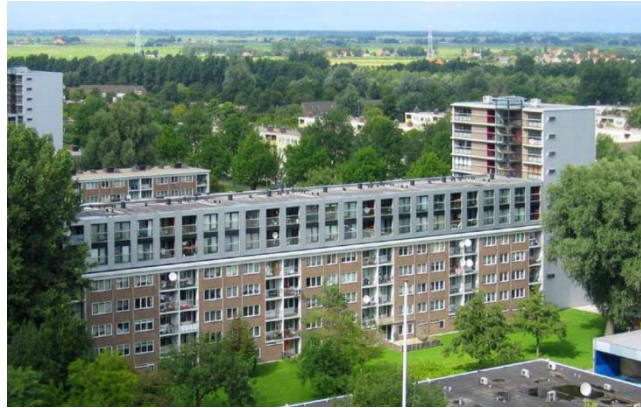
Figure B.11: Top-up realized on a council estate (Duinluststraat) (Hans van Heeswijk architecten, 2003).
