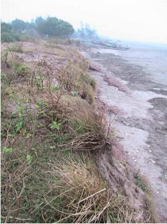
Sea dikes with Vetiver grass on outer slope
