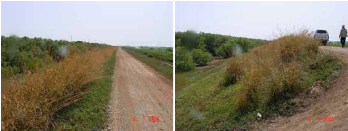
Picture 1-1: Fifteen months old Vetiver on the outer batter of the sea dike in Go Cong province, Viet Nam
