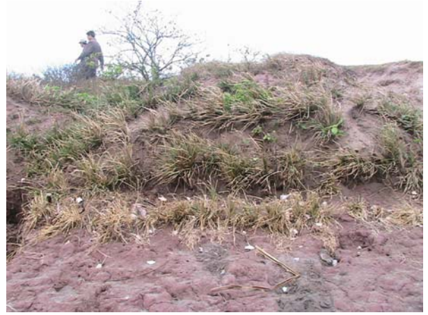
Details of outer slope of Nam Dinh sea dikes with Vetiver grass protected
