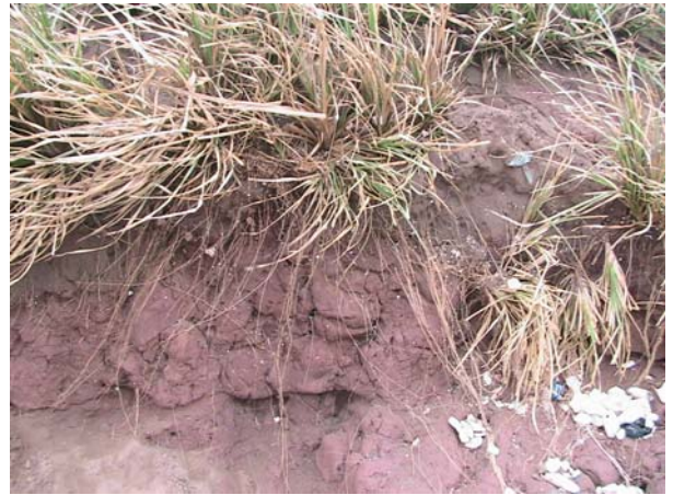
Erosion of dikes slope which has been protected by Vetiver grasses
