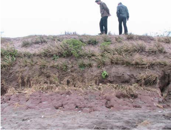
Details of outer slope of Nam Dinh sea dikes with Vetiver grass protected
