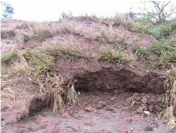
Erosion of dikes slope which has been protected by Vetiver grasses
