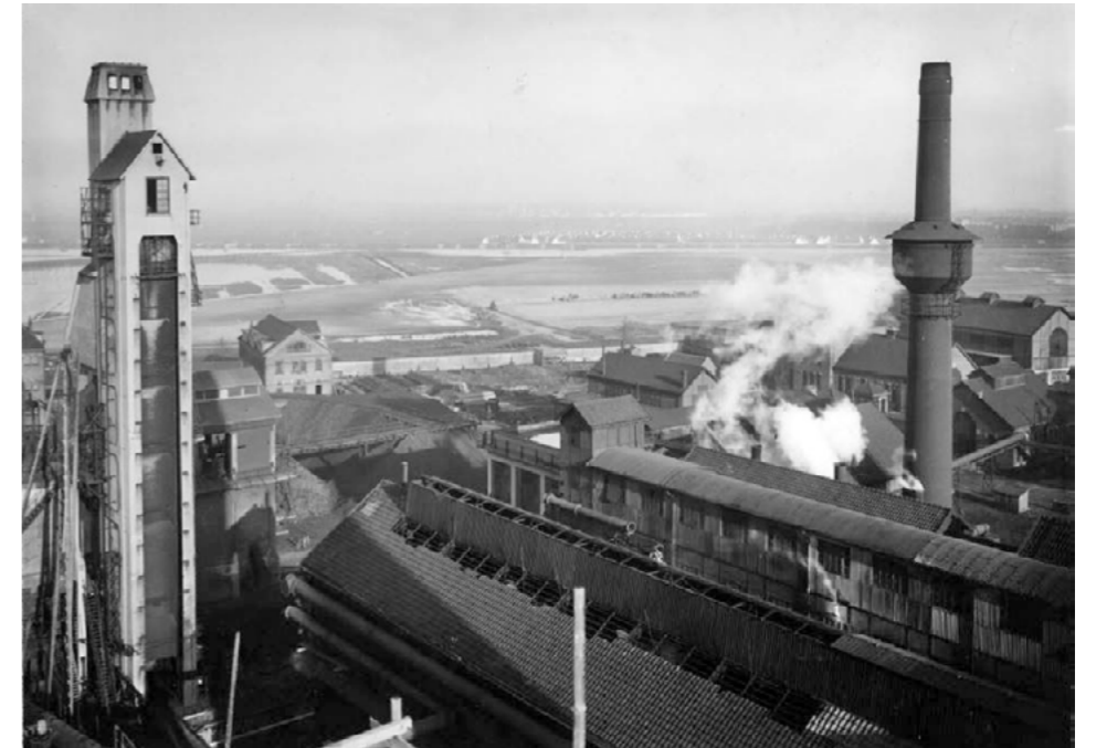
Gas factory Keilehaven 1924
