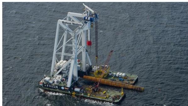
Figure 2.5: Wind turbine foundation installation with the vessel Svanen
