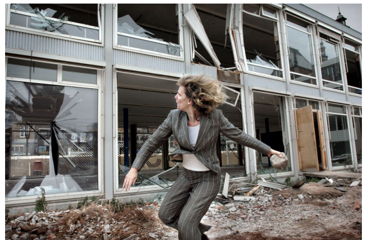
Figure 6, J. van den Broek (2006), Start of the demolition of the Sandberg-wing [Photo].
