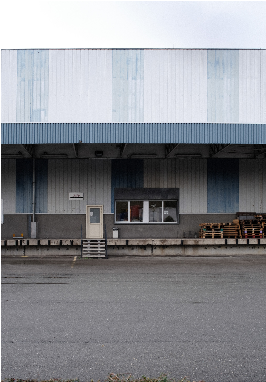
washed out paint
