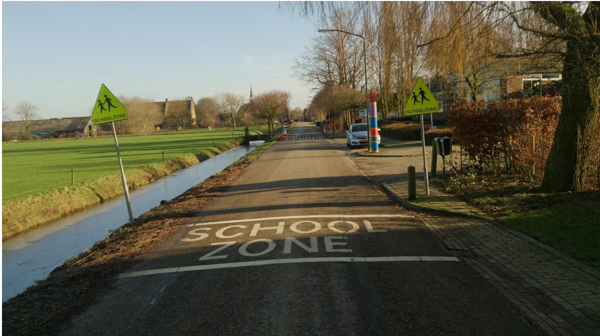
Figure 31: Marking the start of the school zone at the school Den Biekûrf in Babyoniënbroek
