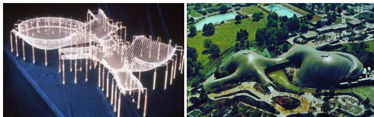
Figure 2: Roof for Multihalle (multi-purpose hall), 1970-1975, Mannheim, Germany
