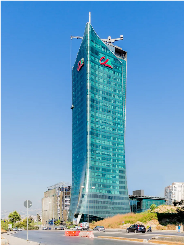
Figure 18. Cold bent glass façade (Credit Libanais beirut, 2013)
