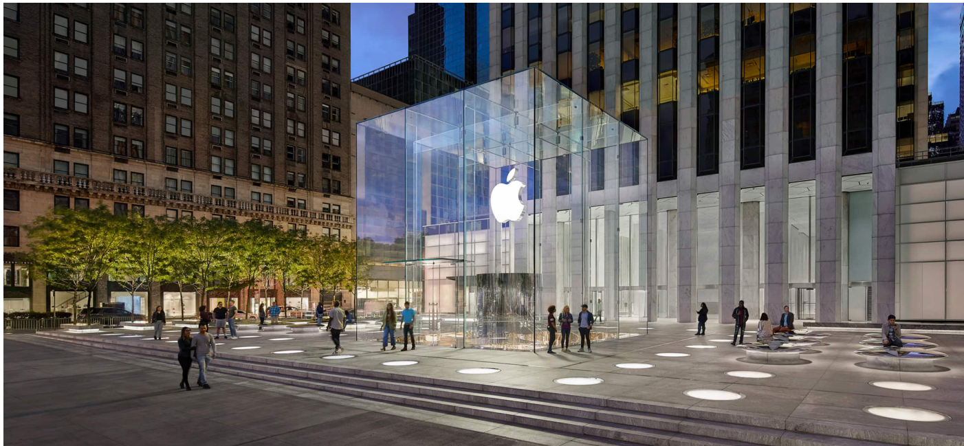
Figure 11. Apple store New York, this picture shows the unmatched transparency a structural glass structure can provide. No big other load bearing
