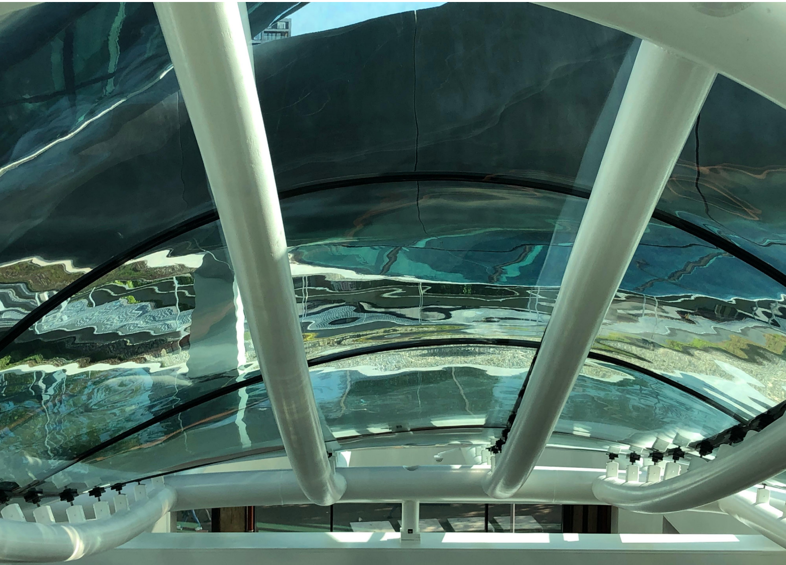
Figure 123. Roof of Fenix Rotterdam made with hot bend panels (Picture taken by author, 2025)
