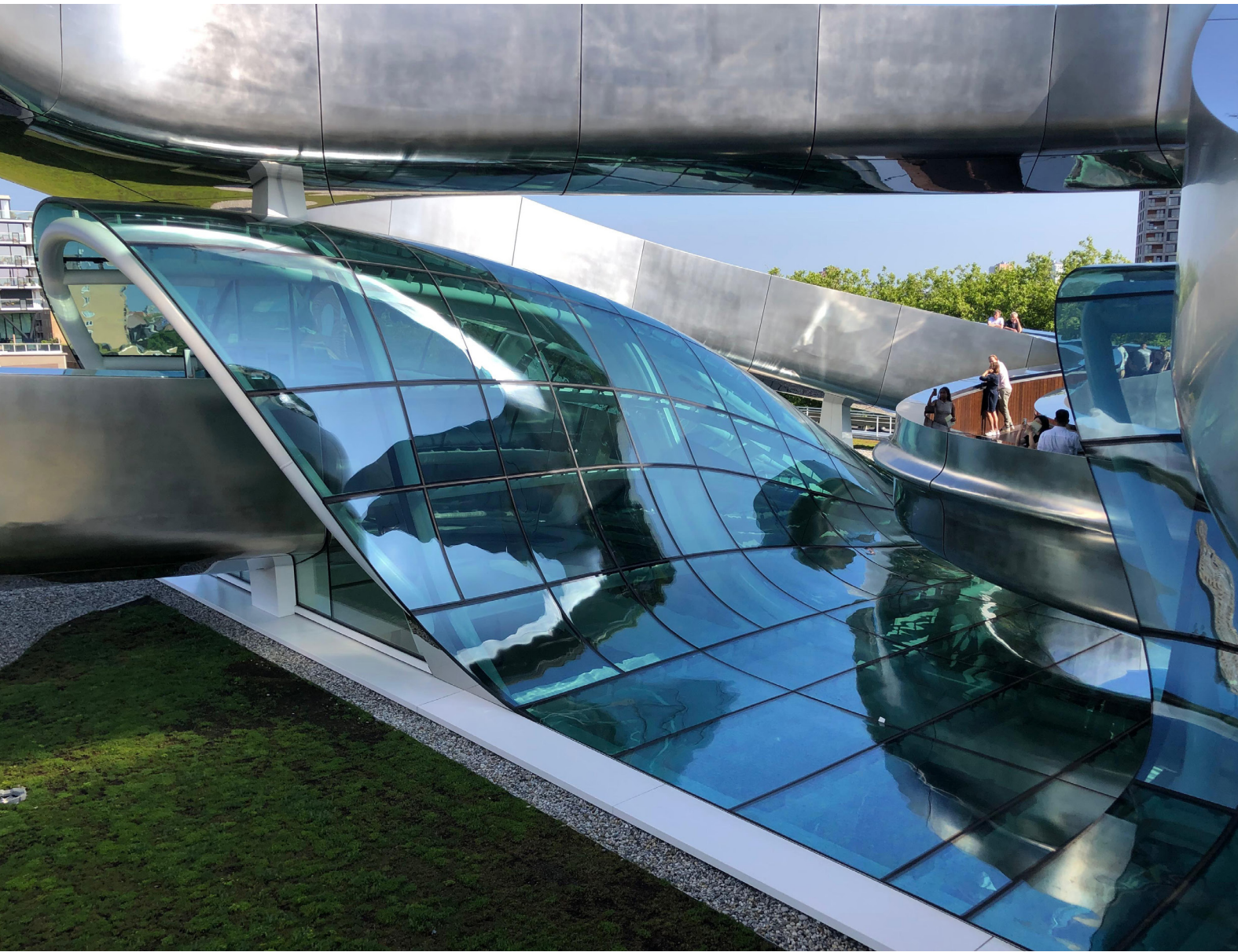
Figure 121. Roof of Fenix Rotterdam made with hot bend panels (Picture taken by author, 2025)
