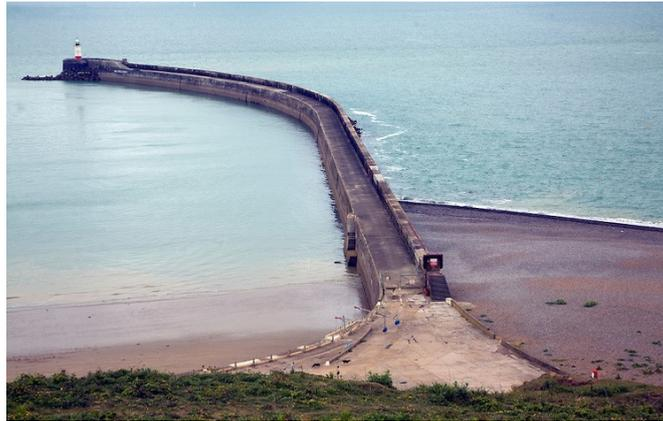
Figure 5.13: Sedimentation around a large concrete groyne in Newhaven, East Sussex, England
