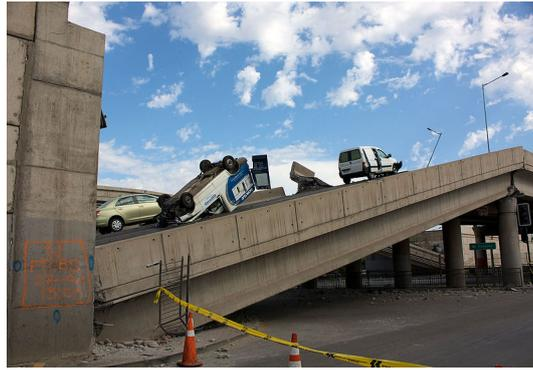
Figure 4.10: Vespucio Norte Express bridge, liquefaction was one of the causes for collapse (Maldonado, 2010).
