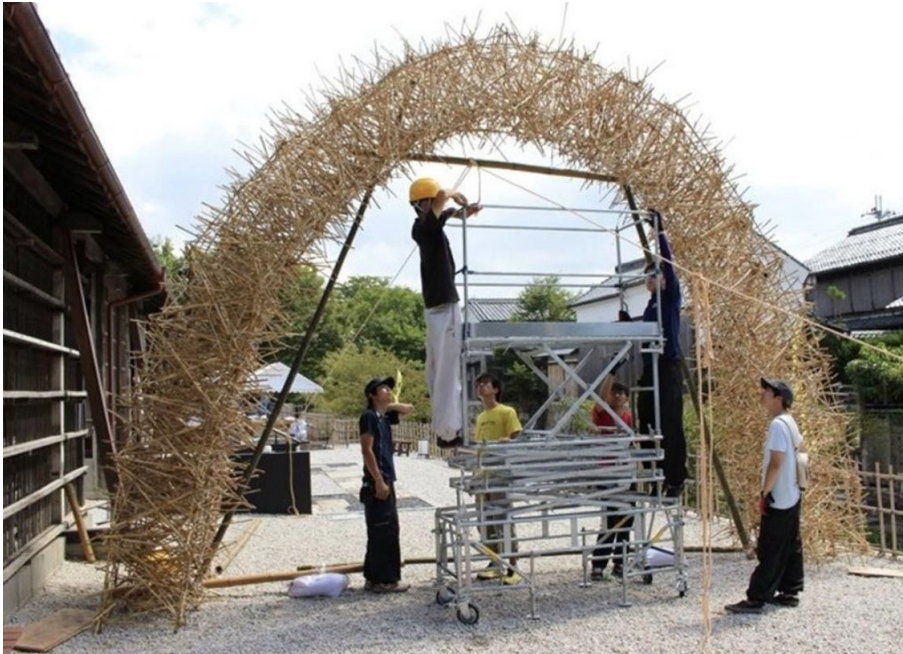
Figure 10: The reed structure is formed from arches consisting of straight, tied pieces of reed. Design and Construction of Temporary Pavilion Using Reed as Structural Material, Japan (Shirai, 2016).
