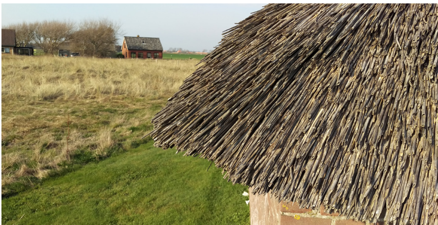
Figure 3: Thatched Reed Roof on Texel Island, Netherlands (By Author, 2019)
