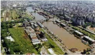
Puerto Madero before works
