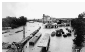
Flood in Entre Rios 1959
