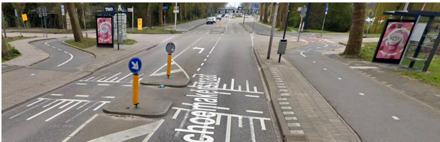
Fig. 2. The observation location was a crossing at Schoemakersstraat in Delft (image: Google Maps Streetview, coordinates: 51°59'52.1"N 4°22'48.3"E). Foreground, at the crossing path indicated by white markings: high curbs with only small cuts (curb is 11 cm on the right, 8 cm on the left). Left and right: bike lanes between sidewalk and road. Side roads from left and right with full curb cuts on their crossings, from which vehicles and pedestrians turn into the road. Background, another main road crossing with full curb cuts. Next to the bus stop on the left there is a curb on the direct route between bike lane and bus stop.
