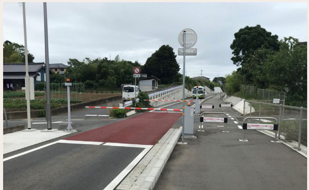
Figure 184. Crossing with existing roads equipped with barriers, Michinori Holdings (2021)
