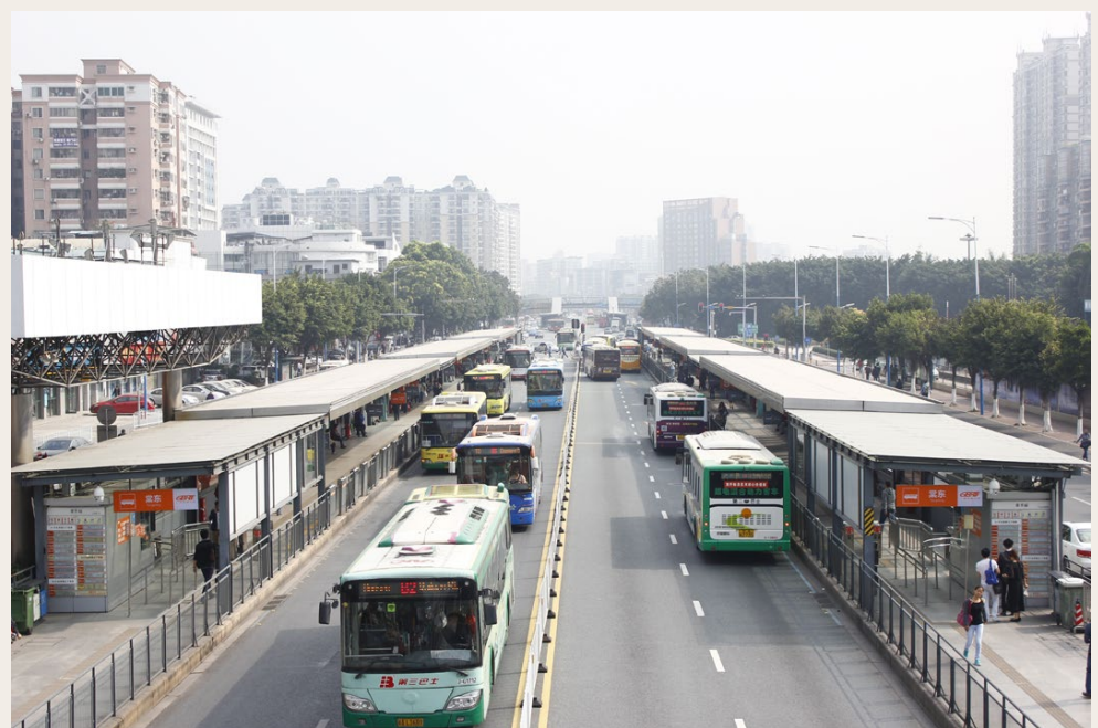
Figure 21. Guangzhou BRT carries 800.000 passengers per day with normal 12-metre buses by operating 31 lines offering direct service leaving and joining the BRT corridor without passengers needing to transfer (Far East BRT Planning Co., n.d.). The stations have dedicated platforms for different lines, and buses can pass each other in the station. Photo taken by the author in 2015.
