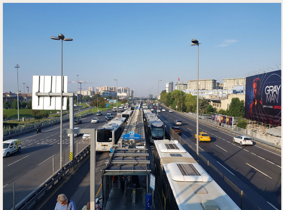
Figure 22. Being the only public transport on land between the European and Asian parts of Istanbul until 2013, Istanbul's Metrobus BRT carries 600.000 passengers per day with 100% articulated buses inside a closed infrastructure (Yazici et al., 2013). There are no passing lanes, and multiple buses stop behind each other every minute. This is the common form of high-capacity BRT in the developing world, which makes it an opposite model of Guangzhou BRT. Photo taken by the author in 2022.
