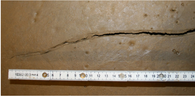
Figure 2.5: Surface depression on the clay surface ahead of a crack.
