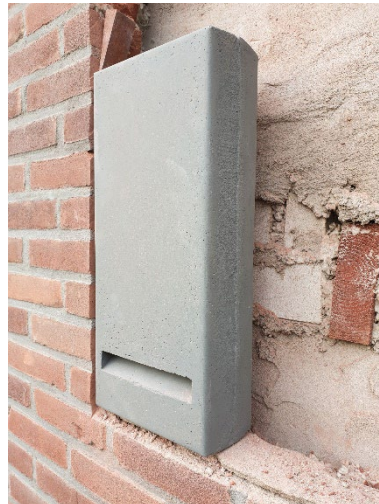
Figure 19. Bat box placed in masonry. Smaller size
