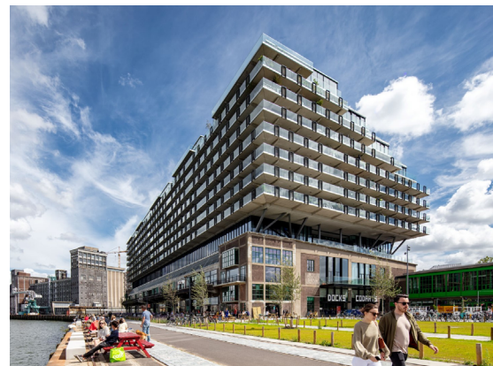
Optimising existing buildings
