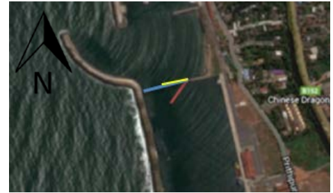
Figure 45: Blockage of entrance cross section by floating breakwater (Google, 2015)
