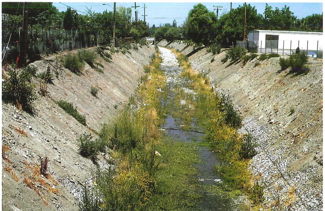
Figs. 24, 25, 26 U.S.A. - California Soil has been introduced into the fill of the Reno mattress revetment to promote vegetation. The box gabion wall however, has been planted-up with suitable plants.
