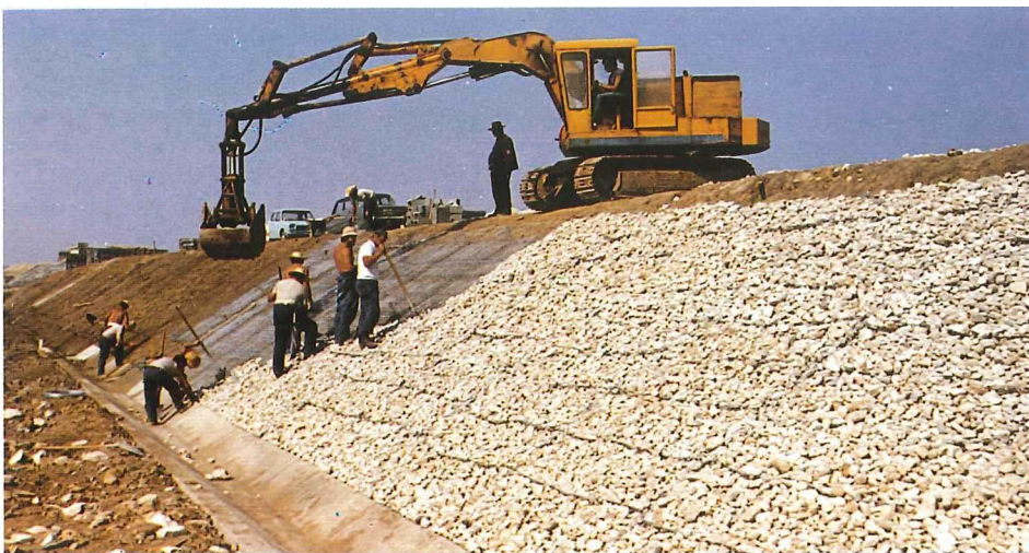
Figs. 52, 53, 54 - ITALY - Lazio Embankment protection with Reno mattresses of the new rail link between Rome and Florence, near Settebagni (Fig. 52). Fig. 53 shows the site some 13 years after completion, showing how the plant growth has restored it to its original state. No such growth has occurred on the same stretch of line where a concrete slab system has been used.
