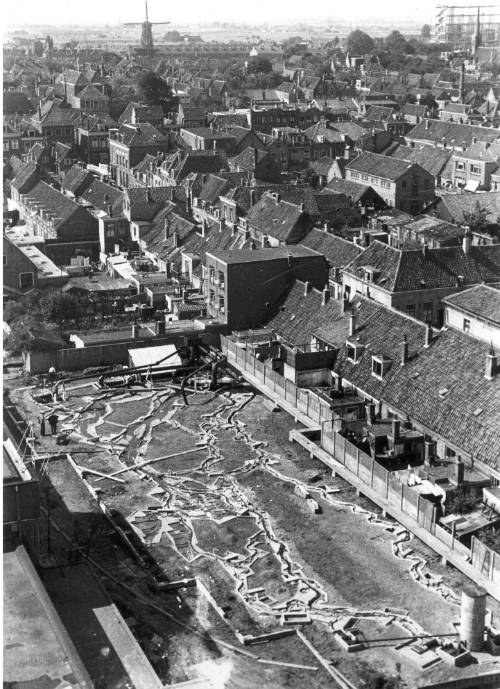
Figure 1.3: Picture of the scale model of the Dutch Rhine-Meuse branches built by the Waterloopkundig Laboratorium in the centre of Delft in 1950. The model was built in the Schuttersveld and the picture was taken from Het Raam. The church on the top right corner is the Lutherse Kerk (also known as Saint George's Chapel) and the windmill on the top left is Molen de Roos. Flow goes from bottom to top. The right-hand branch is the Lek. The second branch starting to count from the right is the Waal. The third one is the Meuse. The upstream boundary is approximately at Wijk bij Duurstede and Tiel. The Biesbosch is visible in the centre of the domain on the left. Picture courtesy of Deltares.
