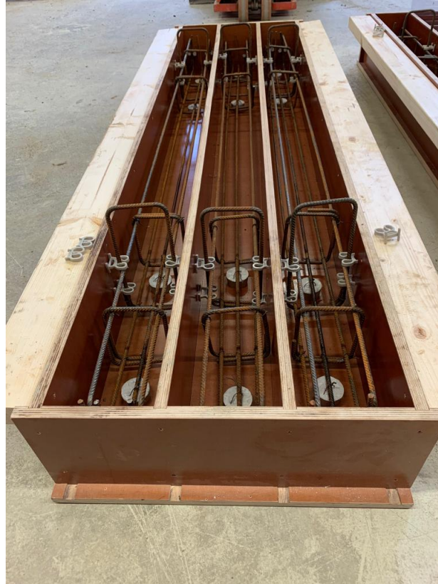
Figure 3.17: Mould for casting along with steel reinforcement
