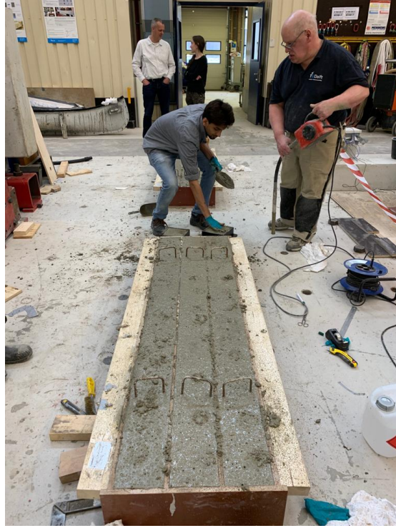
Figure 3.22: Levelling of the top surface of concrete
