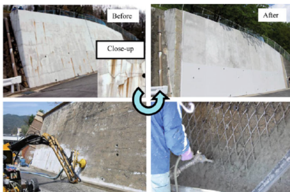
(a) SHCC spray on retaining wall
