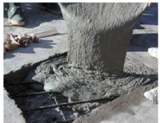
(b) Concrete patch repair
