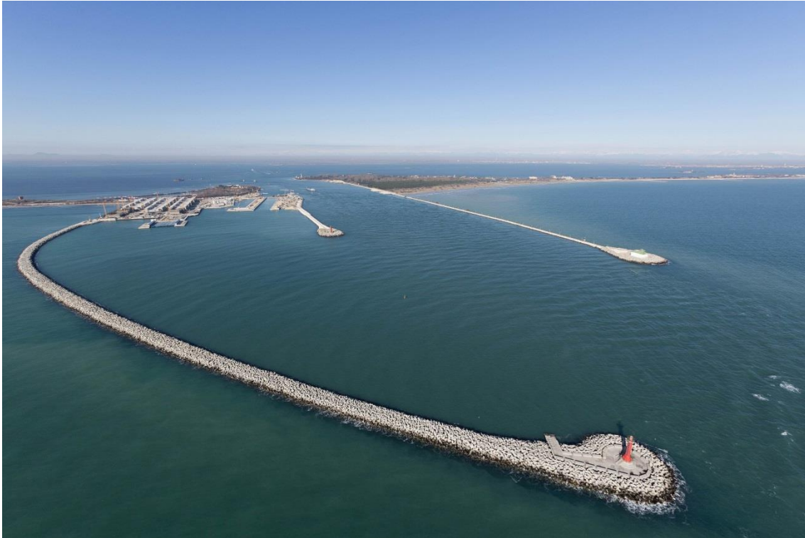
Figure 1.2. Rubble mound breakwater at the Malamocco inlet of the Venice Lagoon ( http://www.salve.it/it/gallery/cantierimalamocco.htm ).
