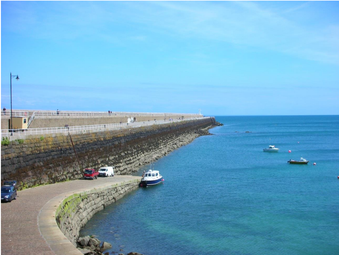
Figure 1.3. Vertical breakwater in Jersey ( http://commons.wikimedia.org/wiki/File:St_Catherines_Breakwater.jpg ).
