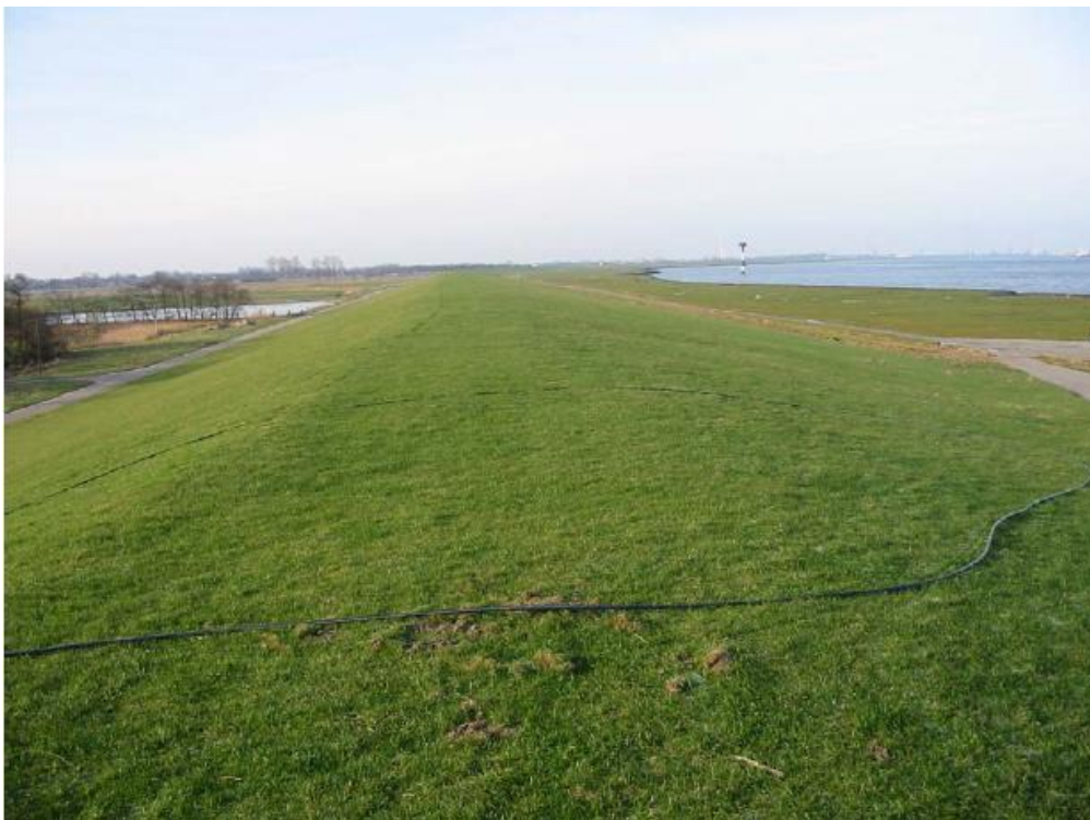
Figure 1.1. Coastal dike covered by grass (source: Eurotop, photo from Schüttrumpf).
