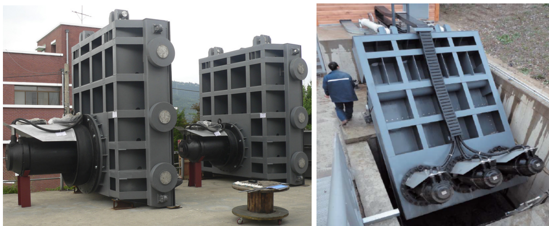
Figure 2.7: Photos of two Hasuh pump gates applied in South-Korea. Noticing the guidance system at the sides of the gate in the photo on the left [12], these are likely to be vertical lifting gates. The photo on the right [13] shows a hinged pump gate.
