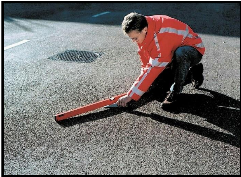
Fig. 2.2 Inspection in progress (CROW, 2011)
