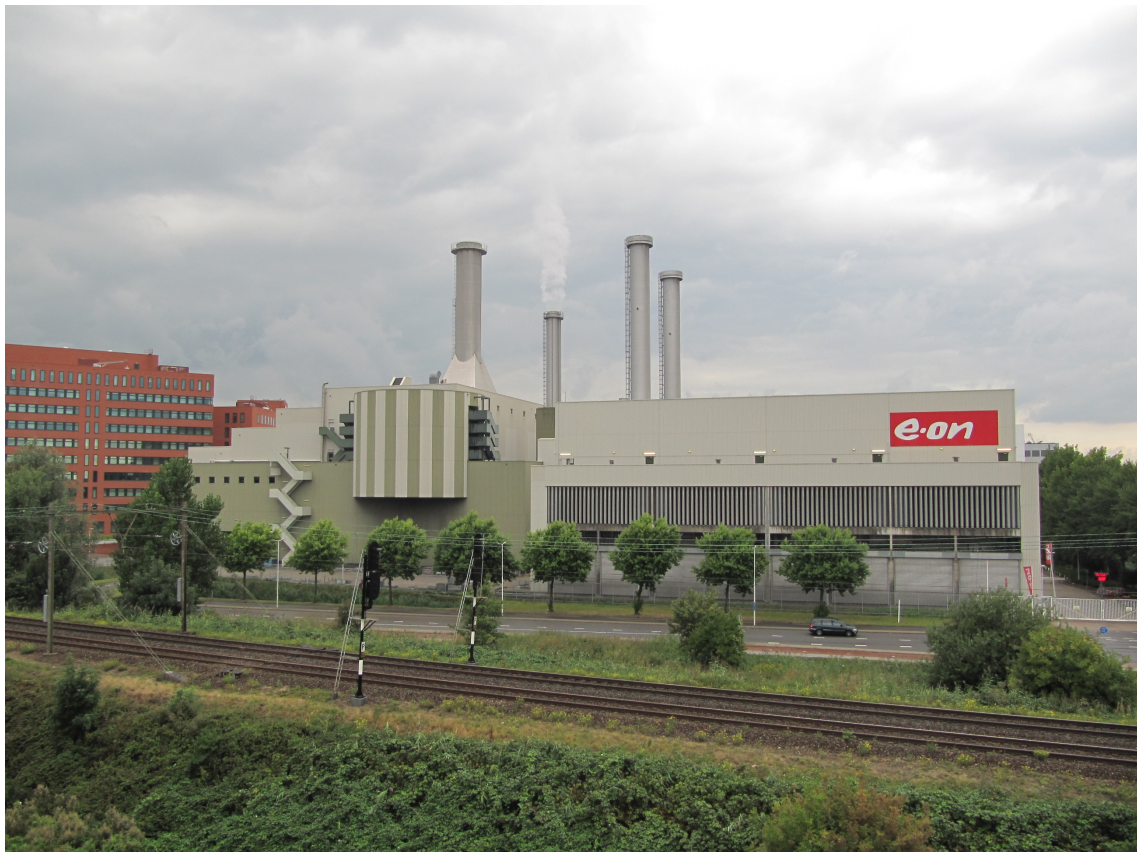
Figure 1.2: Uniper RoCa3 power station in 2013 (E.ON RoCa3 prior to 2016)
