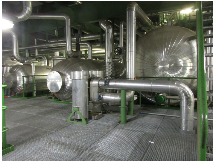
Figure 2.17: Frontal view of the LD drum (left), HD drum (center) and degasser (right)
