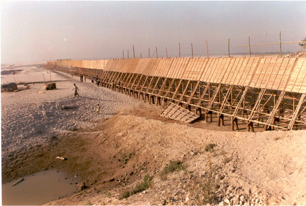
Figure 1 Improved high-water bandals under construction in the Brahmaputra-Jamuna river, Bangladesh
