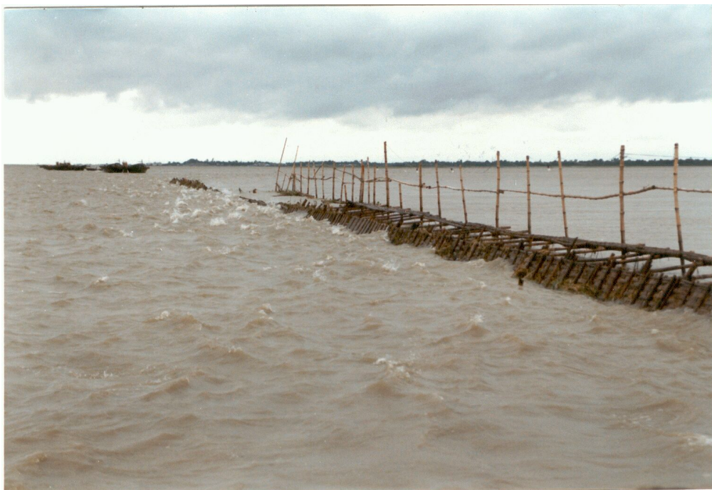
Figure 2 Improved high-water bandals during flood in the Brahmaputra-Jamuna river, Bangladesh.
